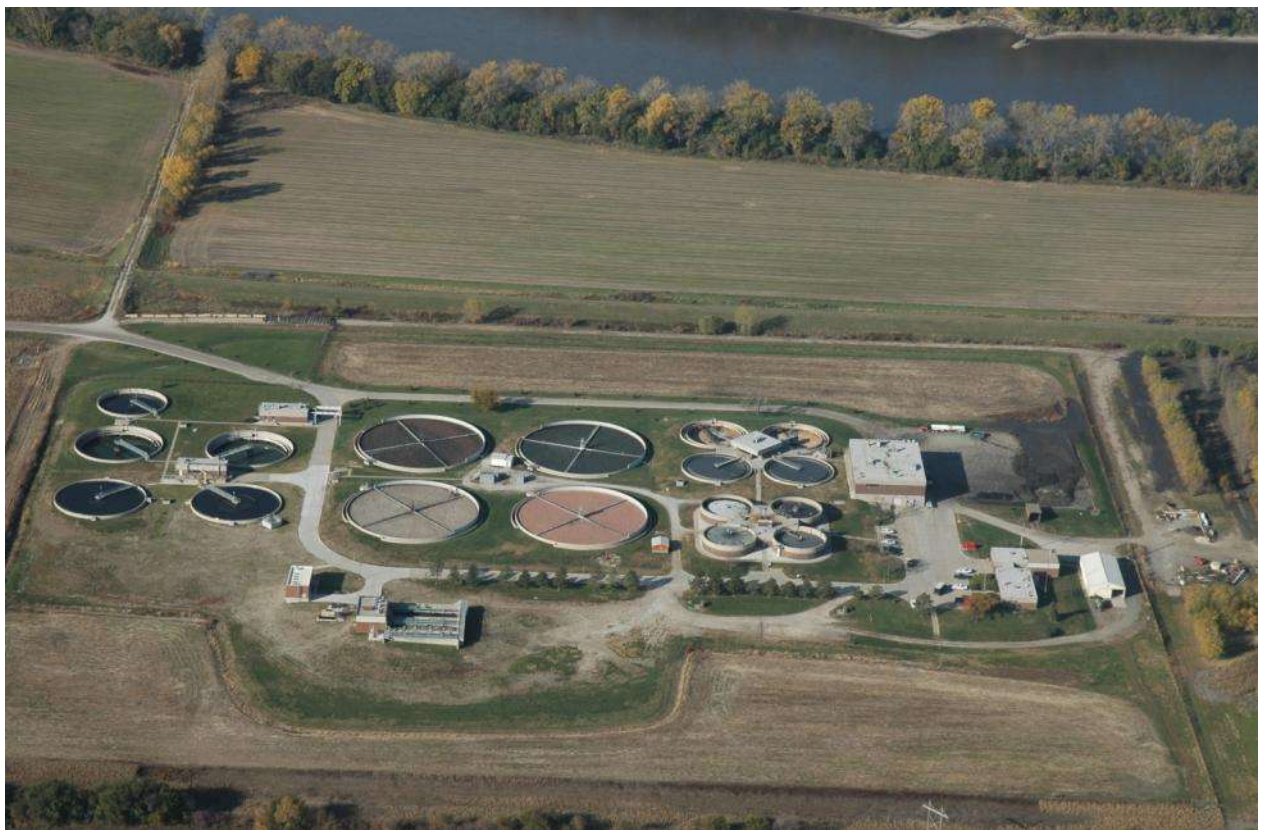
Council Bluffs Water Pollution Control Plant aerial after IFAS construction. Photo illustrates IFAS Basins and new Aeration Basin Influent (ABI) Pump Station in the lower left hand corner as well as rehabbed final clarifiers. Photo also illustrates the Missouri River to the west of the treatment plant. General flow pattern for IFAS system is gravity flow from trickling filters to ABI Pump Station, pumped flow to IFAS Basins and gravity flow to final clarifiers and final discharge to Missouri River.
